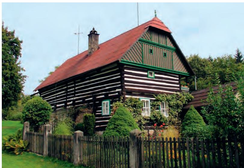
Timbered farmhouse from the end of the 18 th century called „Kopicův statek“. An epitome of vernacular architecture of the Upper Jizera region. Kacanovy, Semily district, Czech Republic. Photo J. Woitsch 2006.
