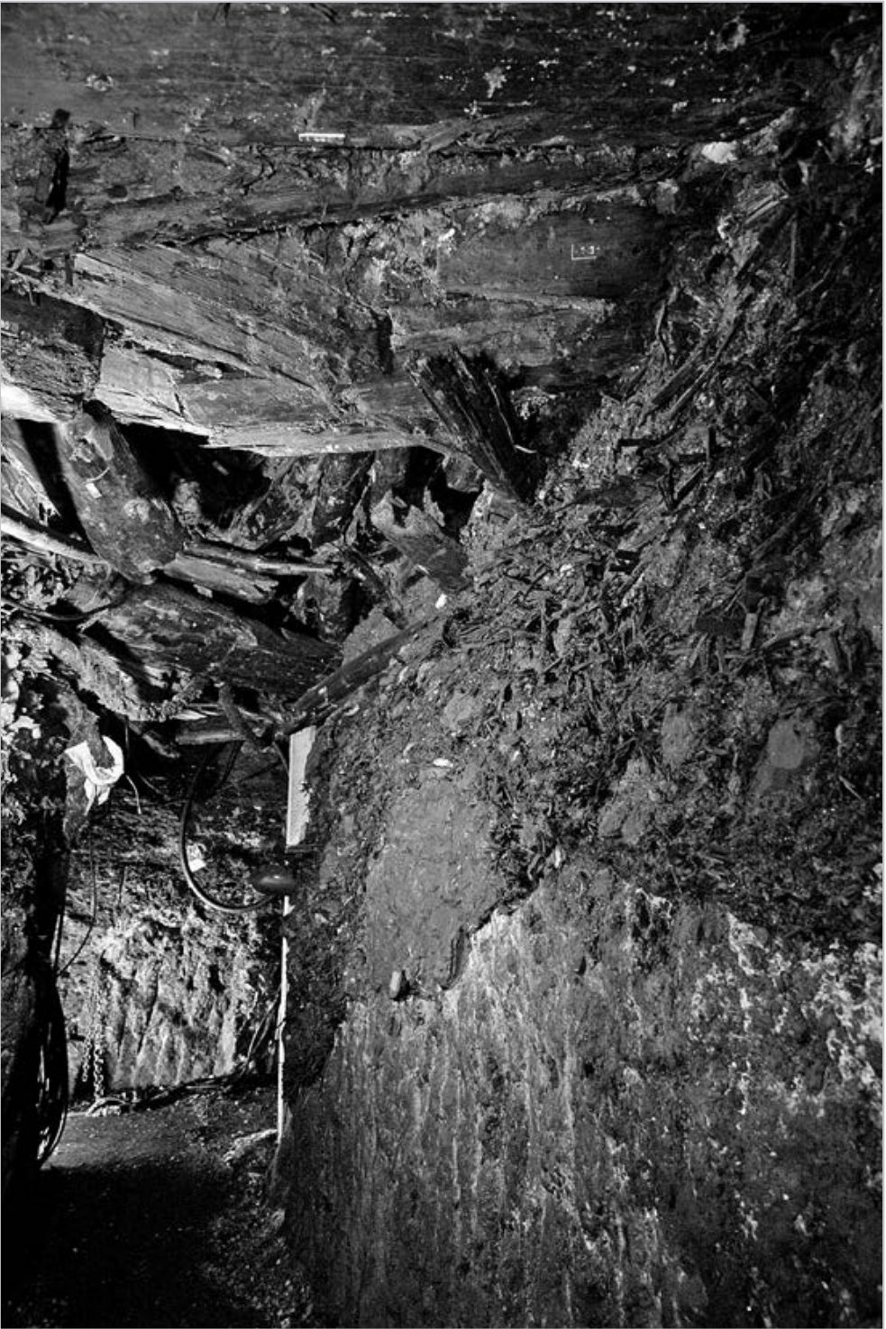
Figure 1: Mine timber at the upper part of the modern tunnel (within the Bronze Age layer of wastes).
